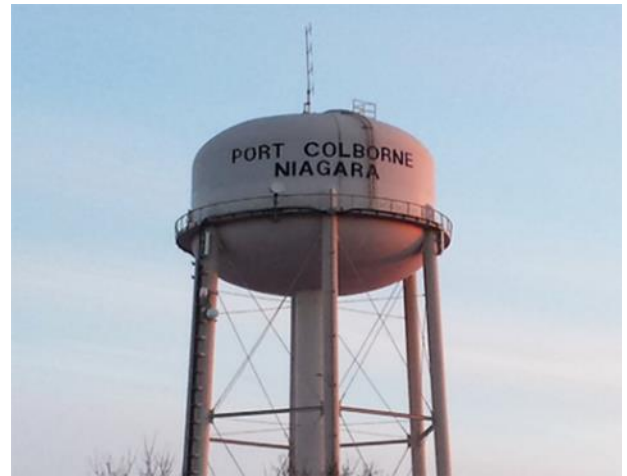
Figure 5: Regional Municipality of Niagara water tower
